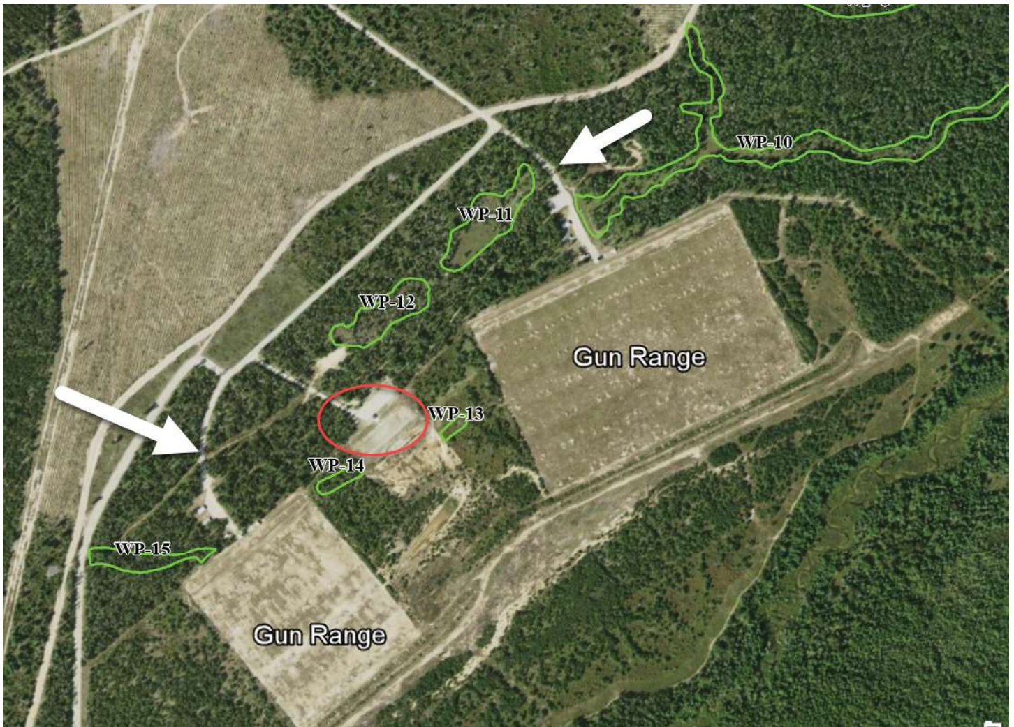
Figure 29. Construction of the gun range resulted in the destruction of prairie habitat. Some infrastructure around the gun range could be modified to mitigate impacts to the prairie. We suggest minimizing roads, especially those that most significantly impact hydrology (white arrows) and creating a central parking area (red circle). Gun range users can park in the central area and walk to the nearby ranges. Removing the roads, ditches, and eastern parking lot would improve connectivity and hydrology of the prairie could be partially repaired. Walking trails from the parking area could function as permanent burn breaks. Mitigating impacts and reversing damages to hydrology of the prairie should be a top priority.
