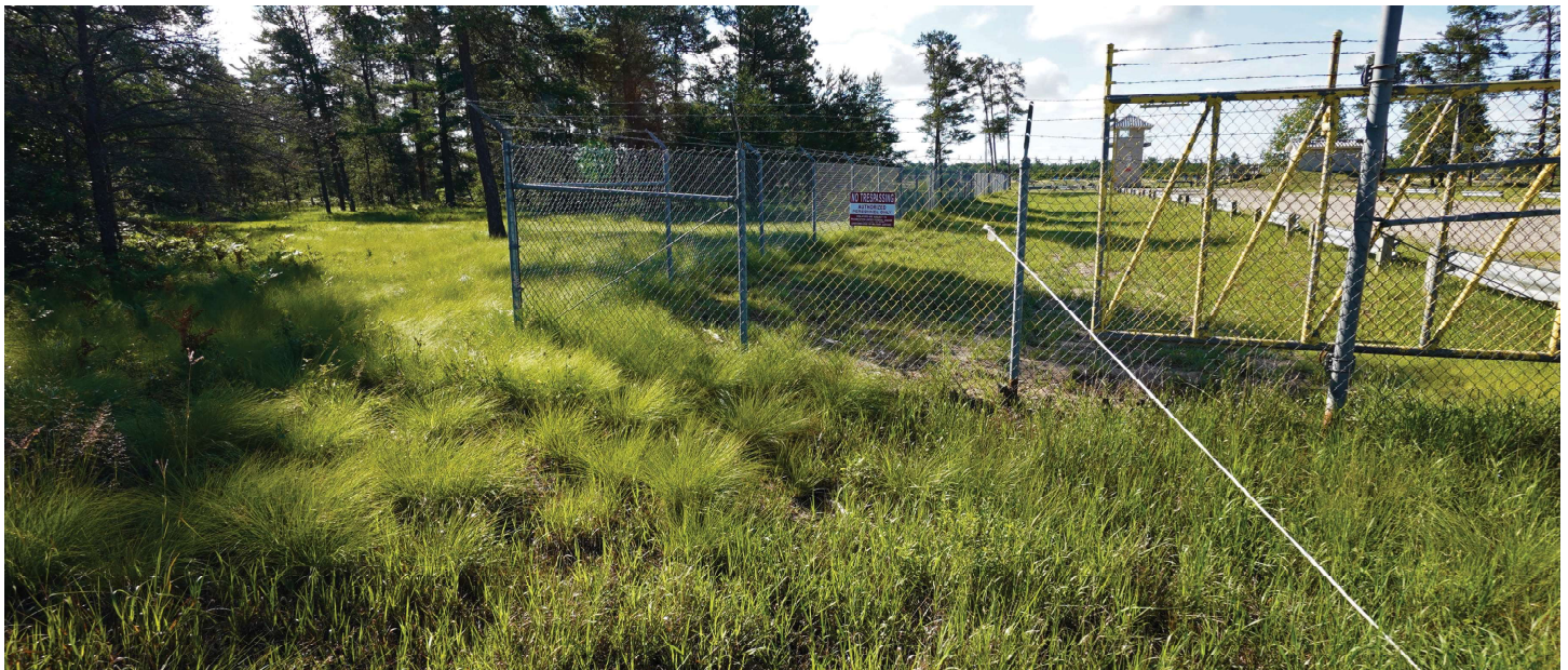
Currently the gun range extends into the prairie. A subtle ditch drains the parking area and the gun range and feeds it into the retention pond.
