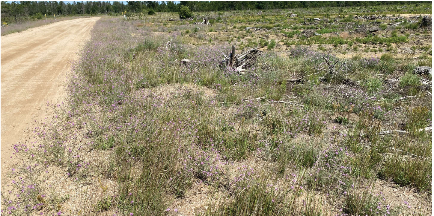
Roads are especially damaging to the prairie because they alter the flow of water through ditching and also act as vectors for invasive species, such as spotted knapweed (pictured above).
