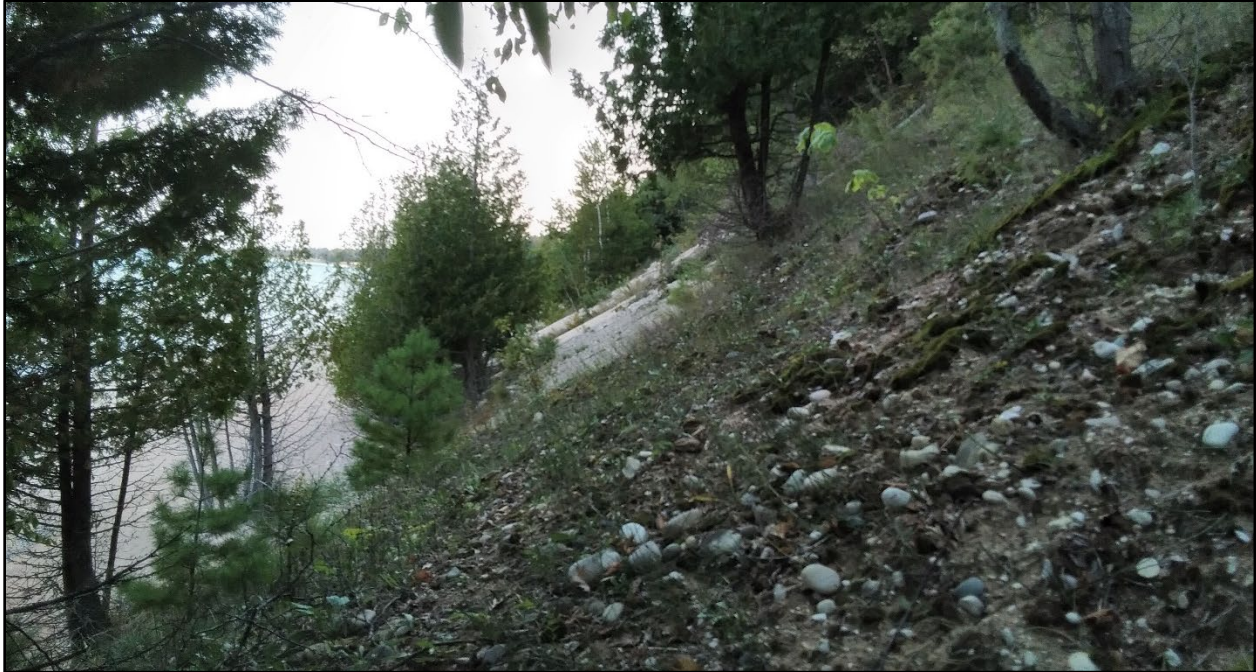
Figure 51. Recent cliff falls can be seen in the steep bluff along the sand and gravel beach (EOID 20444). Photographs taken on September 9, 2022, by Rachel Hackett.
